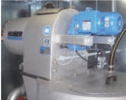
ROTAMAT® Pipe Strainer for wastewater flows of up to 5 l/s
