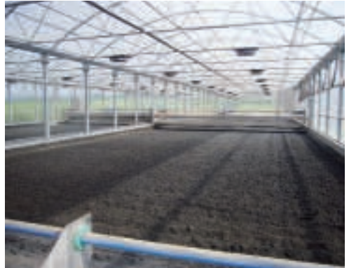
Dewatered sewage sludge becomes dry granulate with the SRT system
