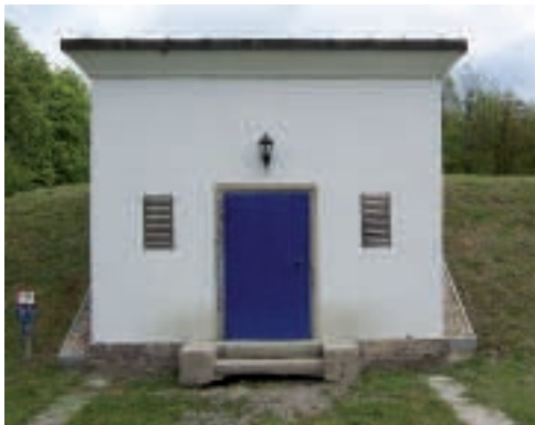
Drinking water reservoir with HUBER equipment
