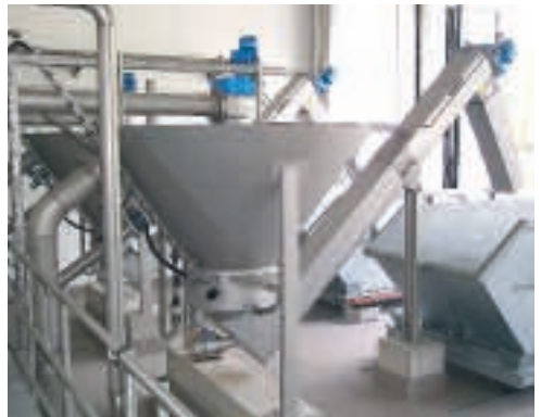
Innovative technology: COANDA Grit Washer RoSF 4
