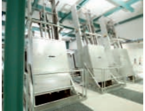
ClimbMax® Screen – a well-proven bar screen for very large flows
