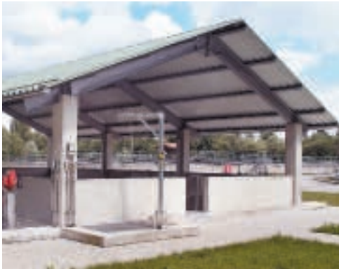
CONTIFLOW® Sandfilter, concrete tank design
