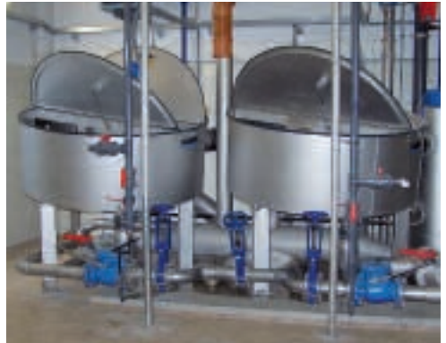
Installation of two units in parallel for WWTP sizes of up to 200,000 PE
