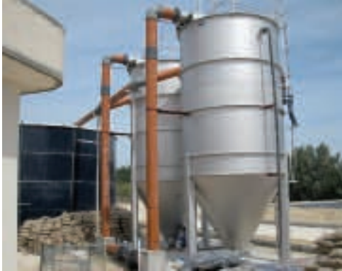
CONTIFLOW® Sandfilter CFSF, stainless steel tank design
