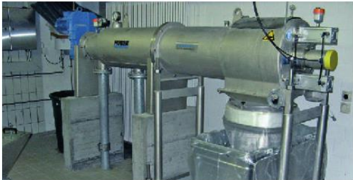
HUBER Sludgecleaner STRAINPRESS® – continuous pressurised coarse material separation
