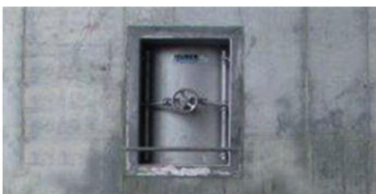
Pressure door, pressure-tight up to a water gauge of 30 m
