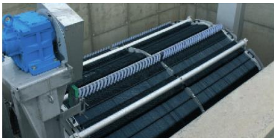
HUBER Membrane Filtration VRM®30 installed in the filtration chamber
