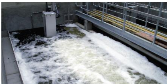
HUBER Membrane Filtration VRM®30 installed in the filtration chamber
