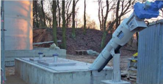
Rotary Drum Fine Screen for coarse material separation installed in an underground tank
