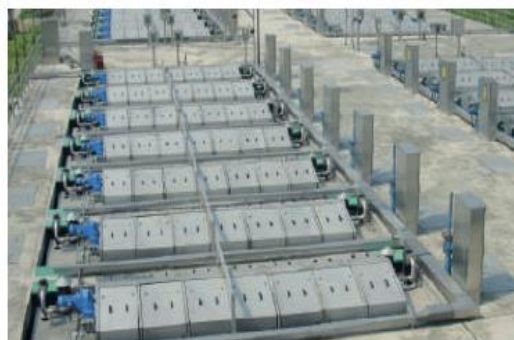
HUBER Disc Filter RoDisc® with up to 35 discs in one unit
