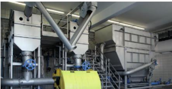
Rotary Drum Fine Screen for coarse material separation installed in an underground tank
