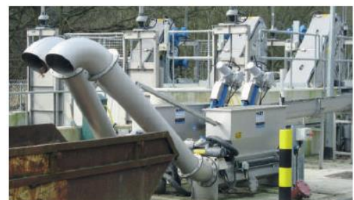
HUBER Wash Press WAP® L with launder channel feeding system: Redundant operation and optimal screenings dewatering
