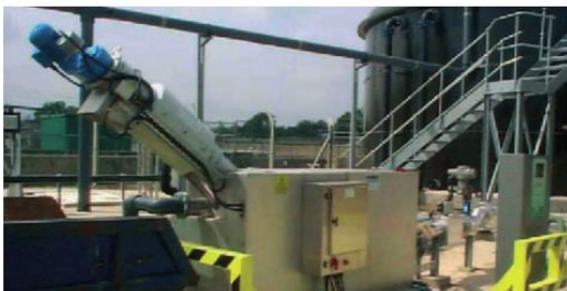
HUBER Sludgecleaner STRAINPRESS® – continuous pressurised coarse material separation
