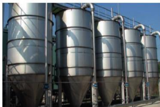
HUBER Sandfilter CONTIFLOW®, stainless steel design
