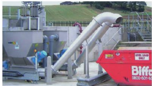
HUBER Wash Press WAP® SL for best screenings washing results
