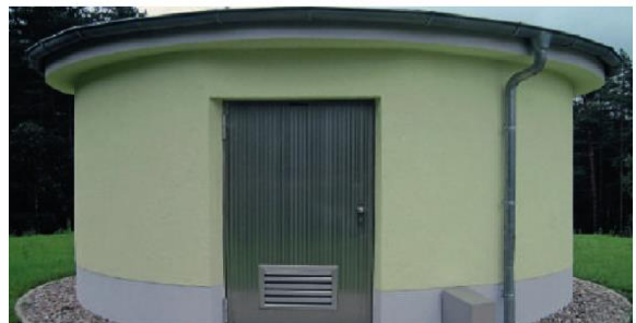
Drinking water reservoir with HUBER equipment
