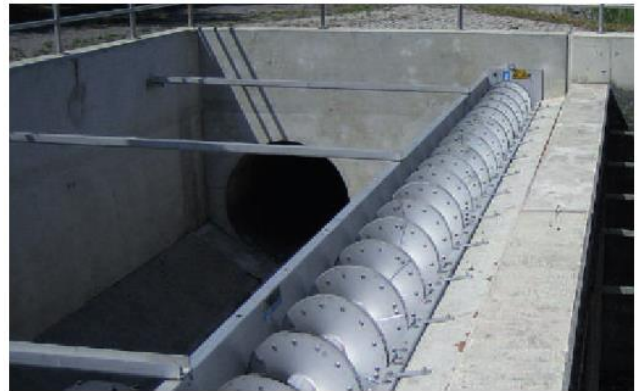
HUBER Storm Screen ROTAMAT® RoK1 installed on dry side of overflow weir
